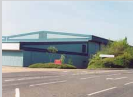
Modern cold store development
